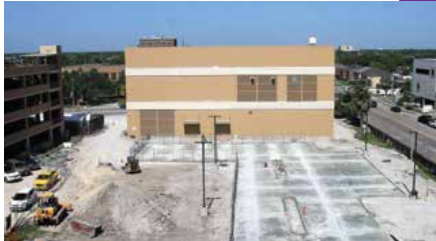
Elizabeth Street Parking lot being poured.
